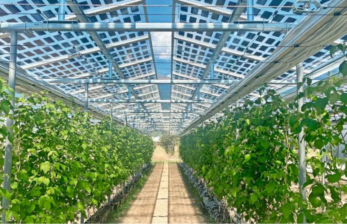
Agri-PV-Anlage in Conthey.
